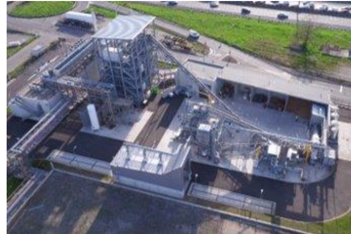
GAYA R&D demonstration plant - St Fons/Lyon – France
